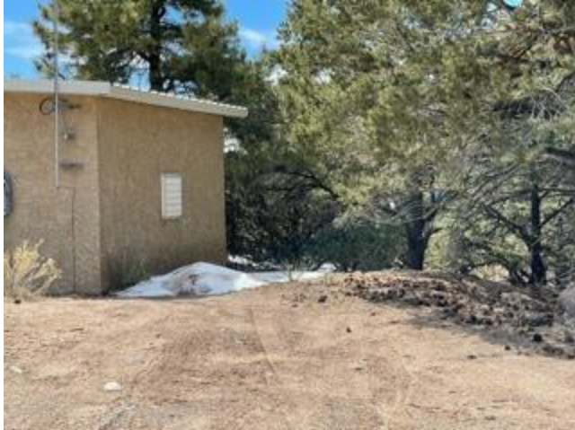
Pine Cone Boost Station: Brush mitigation desirable.
