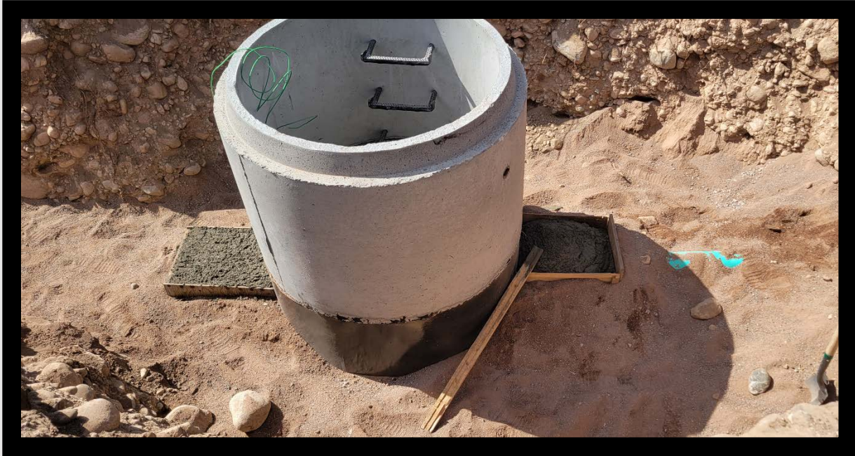
New manhole being installed on Lovers Way 4/28/22.
