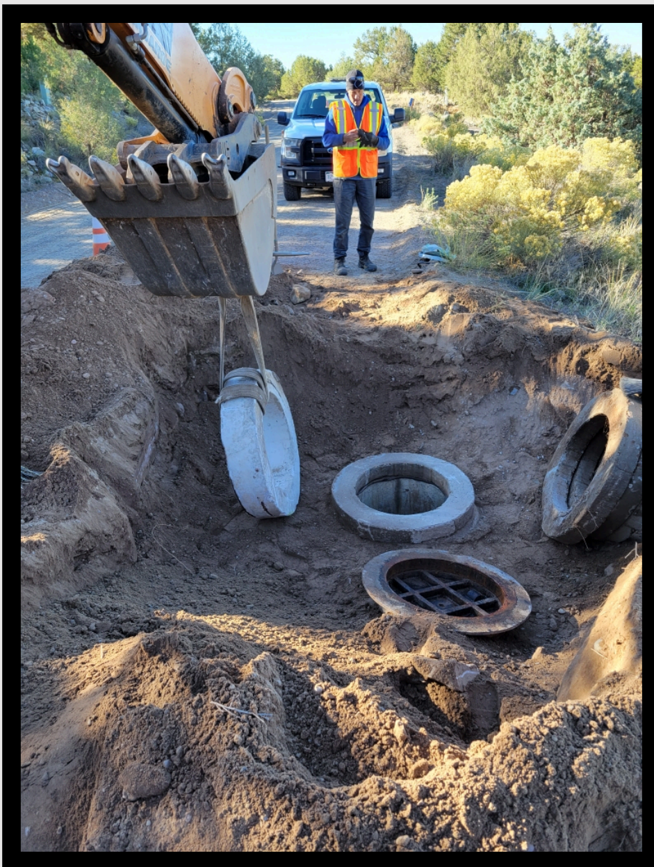
Manhole Lid being raise on Lone Pine Way
