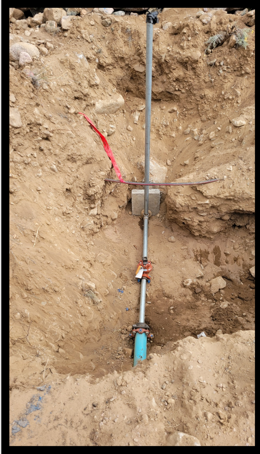
Flushing Hydrant Replaced on Rockaway Overlook
