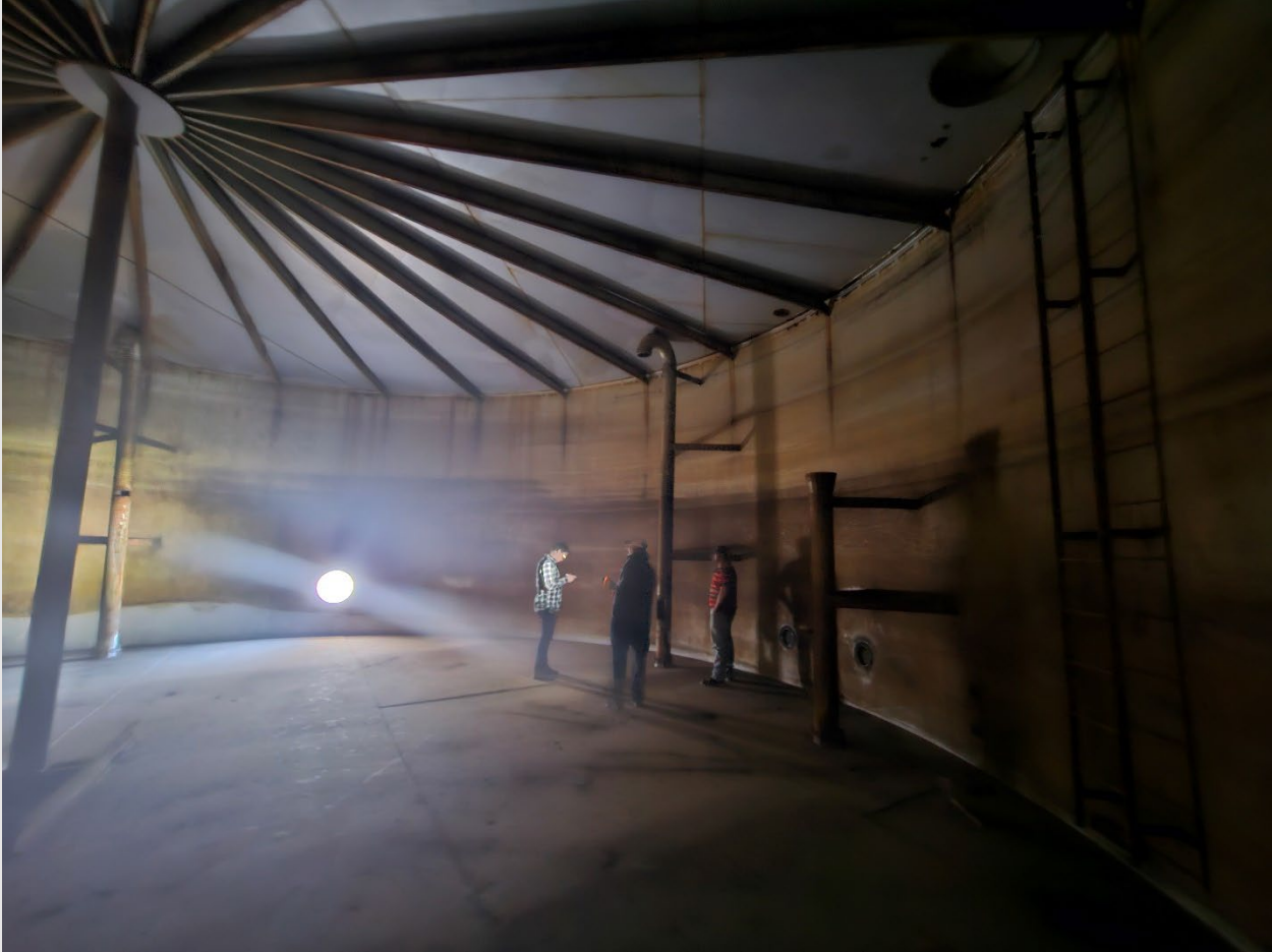
Inside of MHE Water Storage Tank
