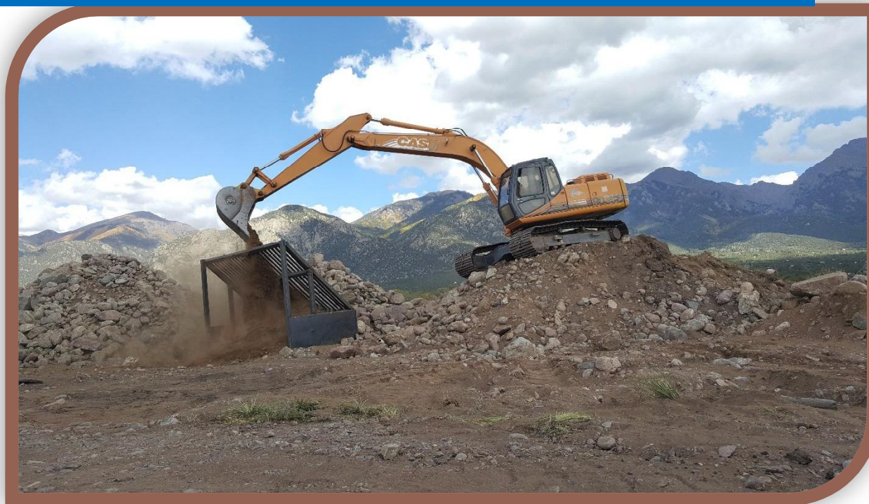
Screening spoils into useful material.
