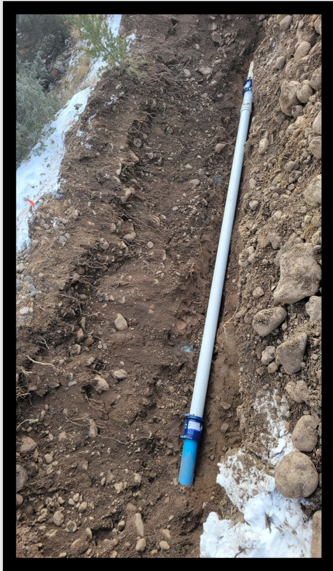
Repaired water main on Spanish Creek
