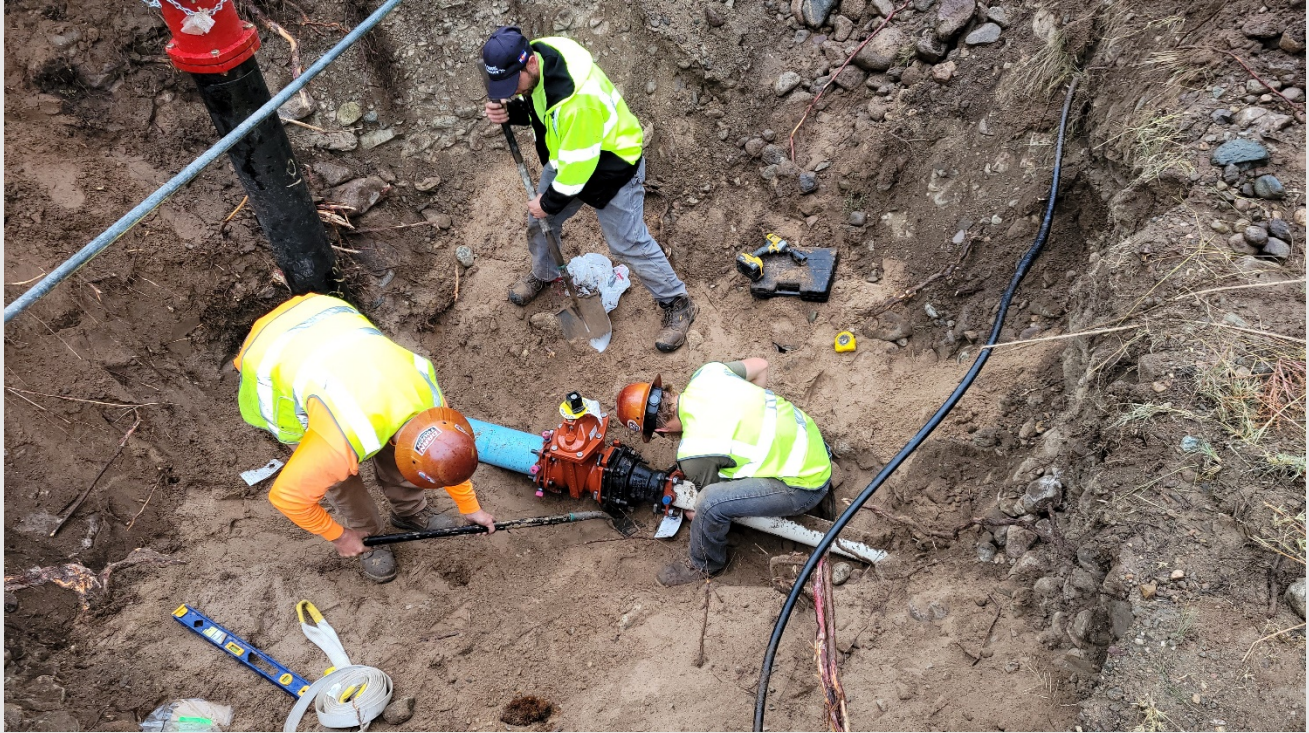
Picture fire hydrant replacement on Willow Creek Way
