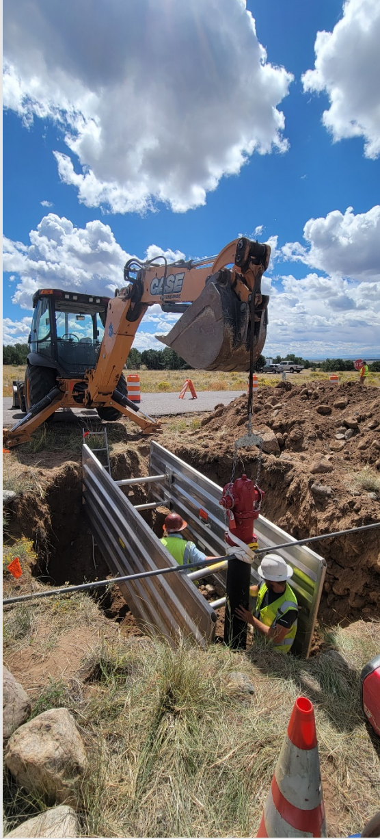
Fire hydrant replacement on Camino Del Rey
