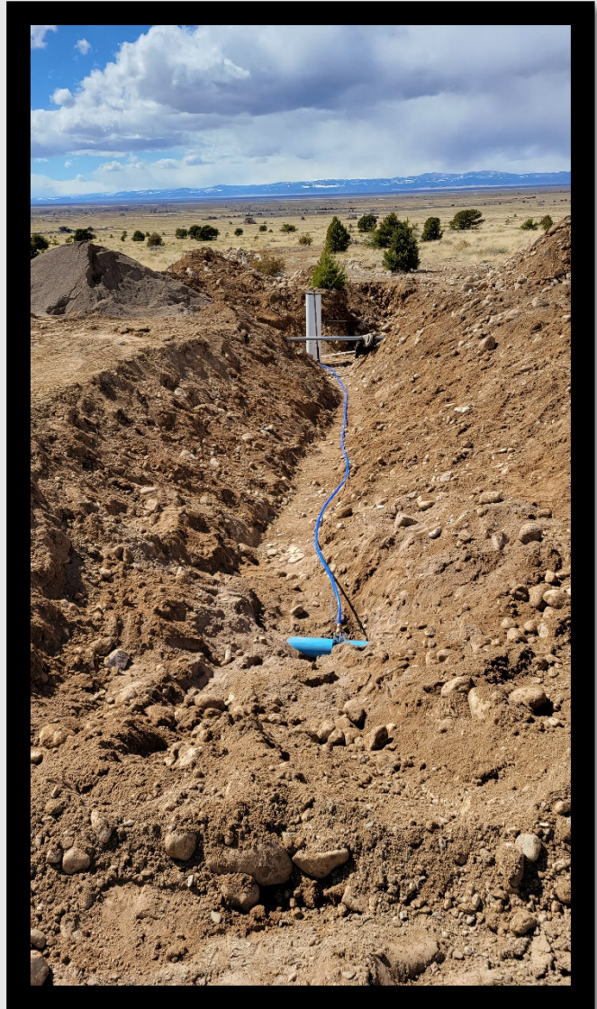
New service line installation 3372 S. Carefree Wav.
