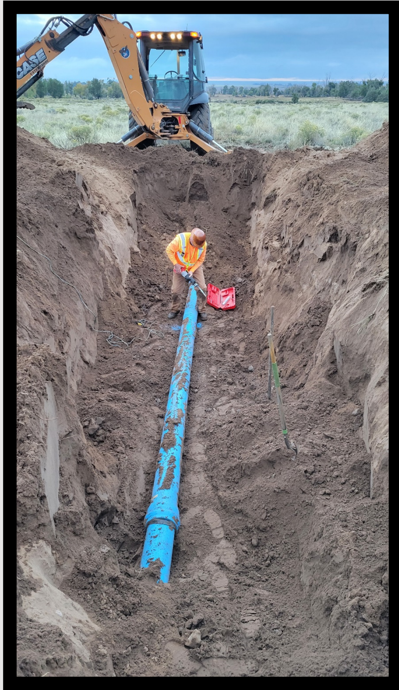
Mark Elliott cutting into broken transmission line
