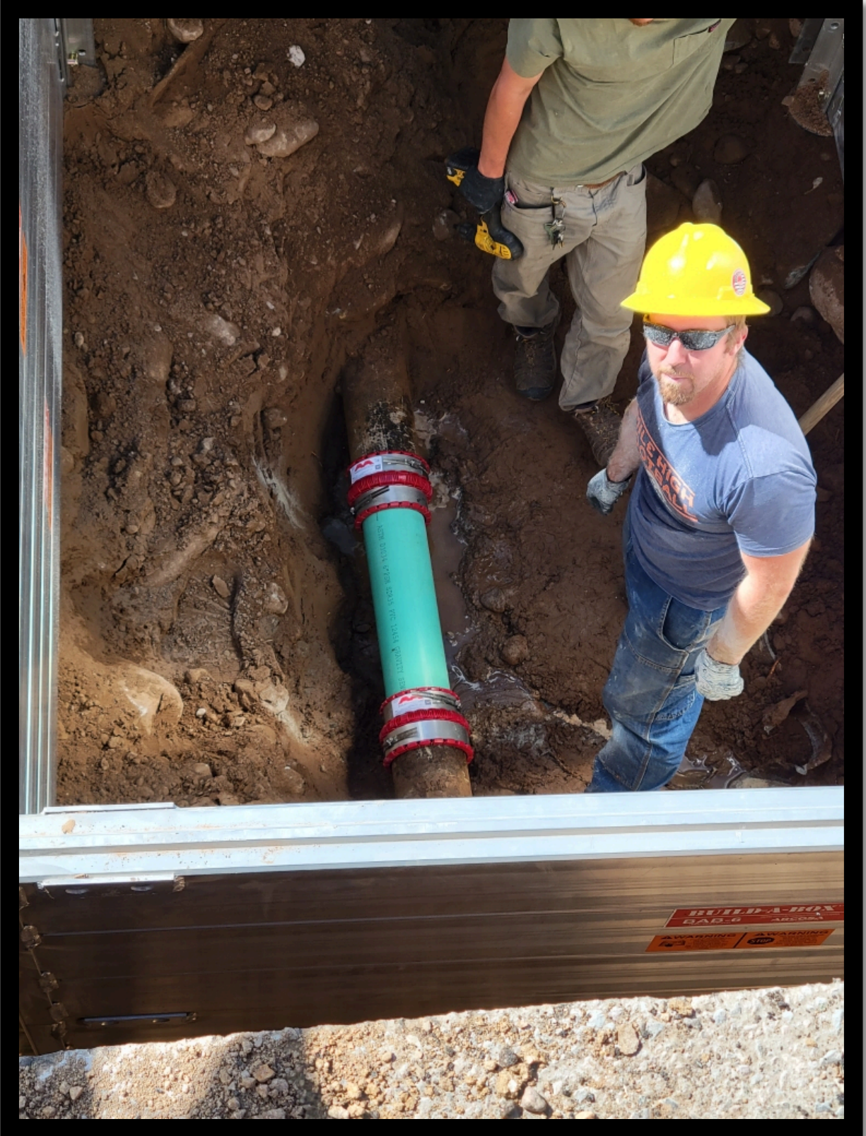
Sewer Main Line On Camino Del Rey After repair.
