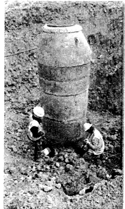
Cottonwood manhole infiltration prevention project
