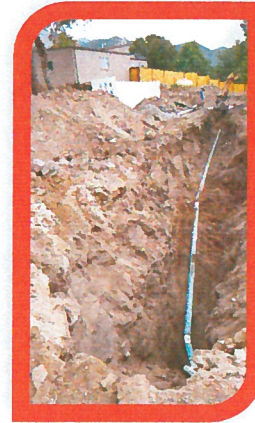
Sewer Service Install
