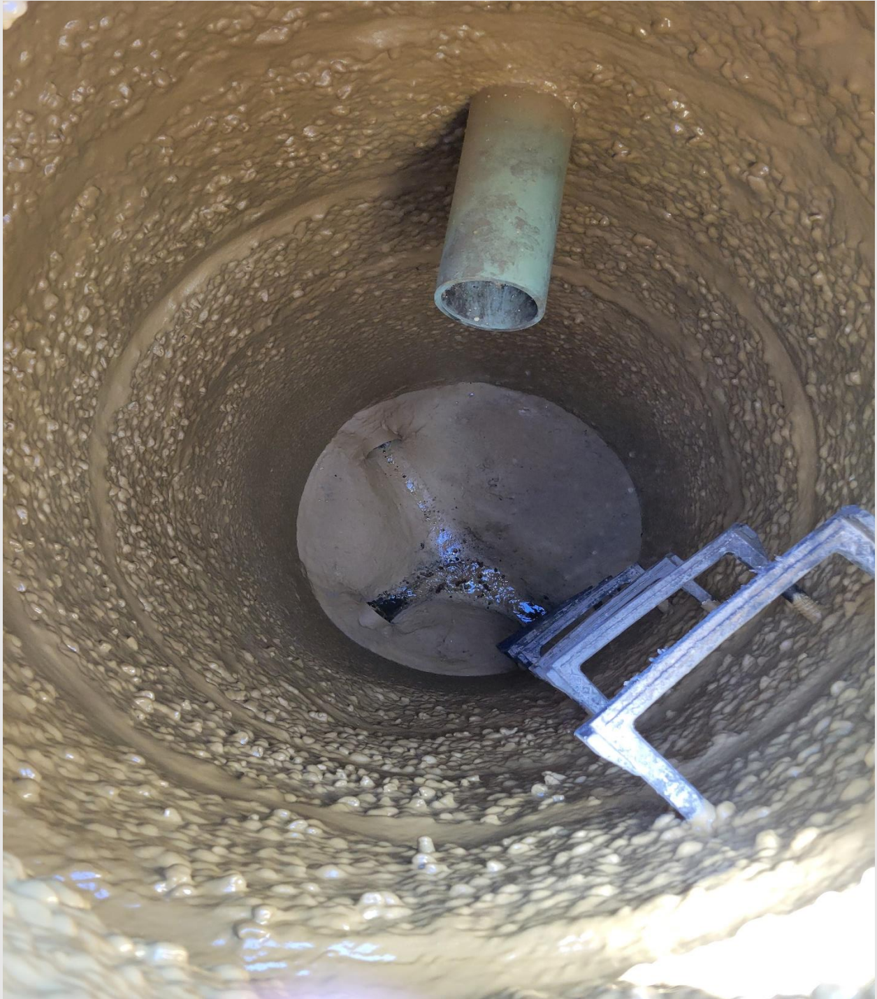
Spanish Creek Manhole after Rehabilitation
