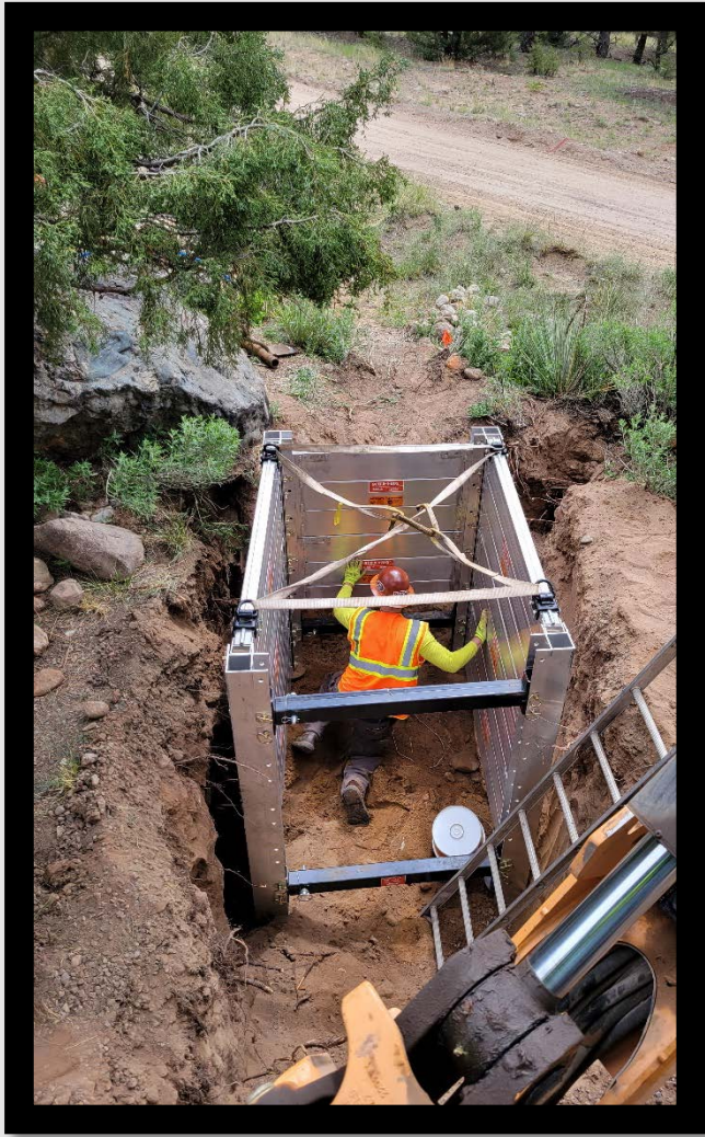
Pictures of new Shoring Equipment being used to replace a meter pit.
